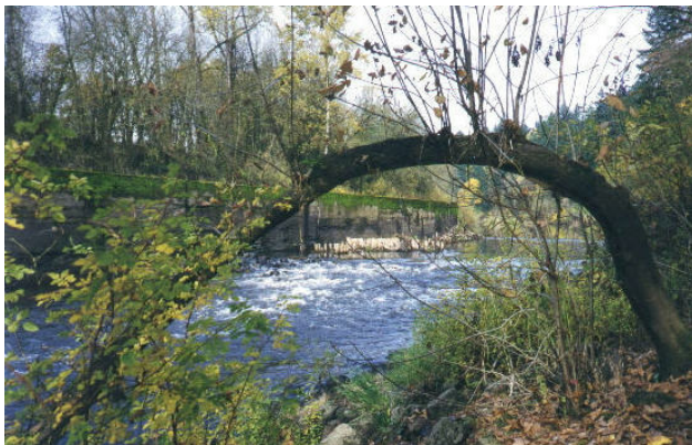
Concrete lock walls at Lafayette Locks County Park [Photo: Yamhill County Parks]
