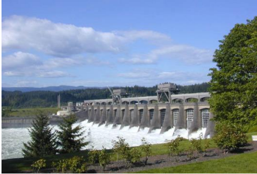
Bonneville's spillway features 18 gates
