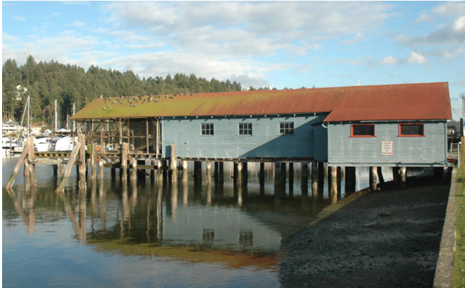
Skansie Netshed dates from 1910 [Photo: City of Gig Harbor]
